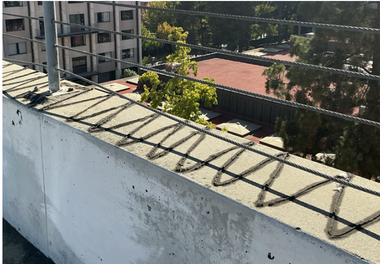
Example of sticky application: applied correctly, but covered in dust over time and diminishing the aesthetics of the facade. .
