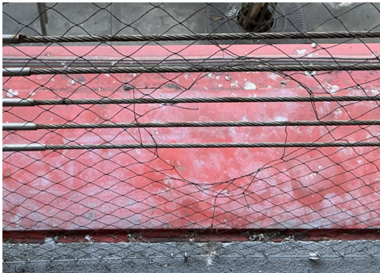
Example of hole in nylon netting.
